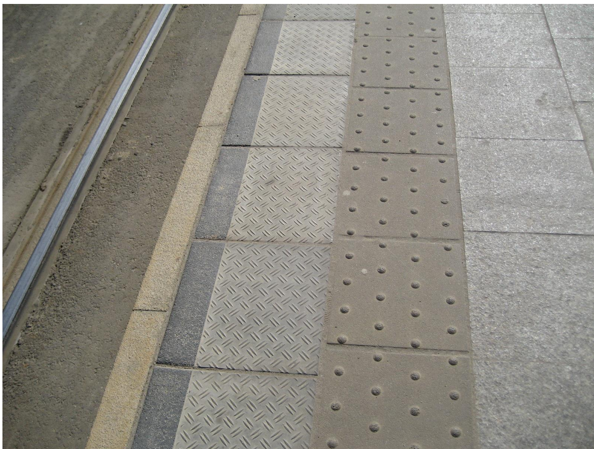
Figure 1. Examples of markings the edge of the tram platform in Warsaw taking into account the guidelines of the Polish Association of the Blind
